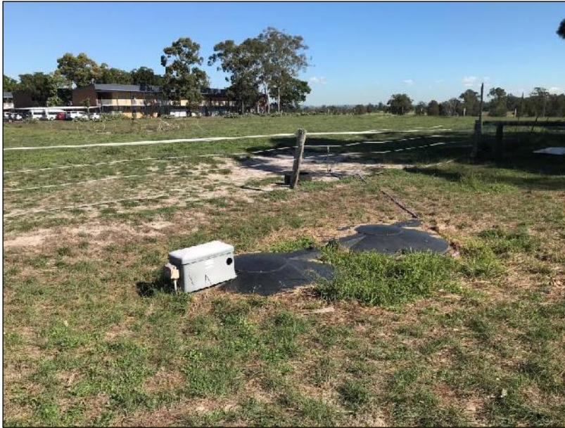
Figure 6: Septic System (Secondary Treatment) with purple hose for irrigation to paddock in background (Landform 1)
